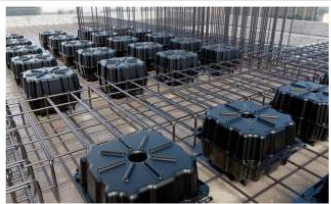
HOLLOW-TILE FLOOR SLABS
